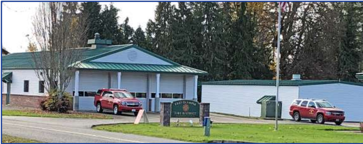
Figure 245: East Olympia Storage & Maintenance Facility (adjacent to Station 61)
