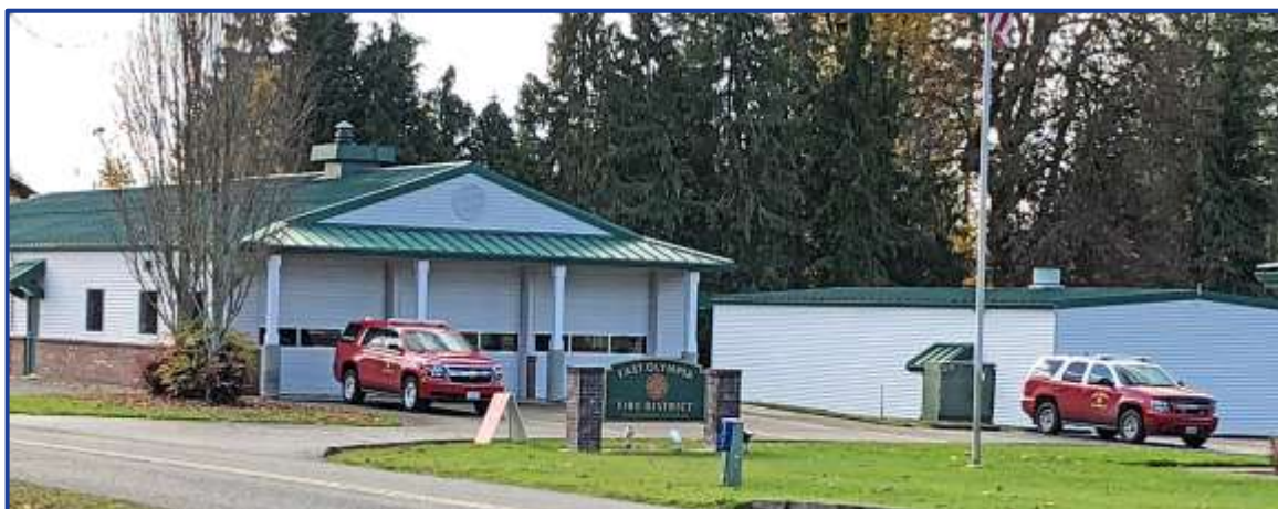
Figure 4: East Olympia Storage & Maintenance Facility (adjacent to Station 61)
