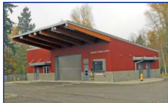
Figure 119: OFD Command Training Facility
